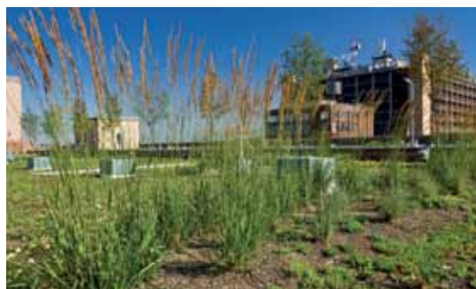
The USPS's new green roof in New York
