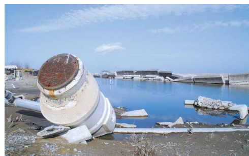
The vicinity of Tsurushihama Beach Resort, Shinchi Town, Soma County, Fukushima Prefecture The manhole that was set in the ground was completely thrust aboveground by the effects of the earthquake. The tsunami washed away most of the buildings in this area as well.
