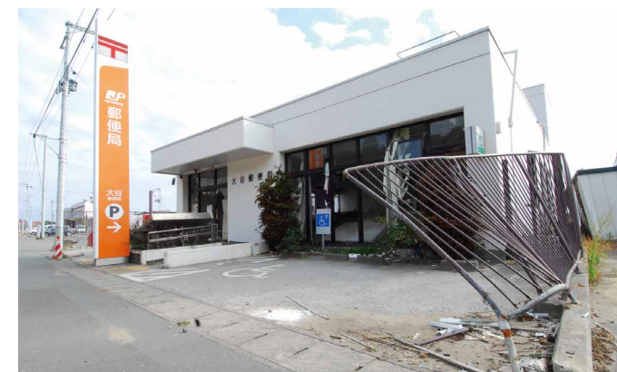
Otani Post Office in Kesennuma City, Miyagi Prefecture This iron fence was severely deformed by the flow of the tsunami.
