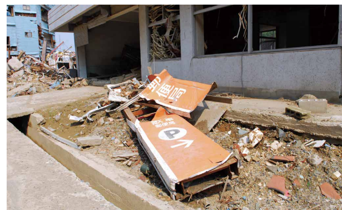
Utatsu Post Office in Minami-Sanriku Town, Miyagi Prefecture This signboard was swept off its base and snapped in two.
