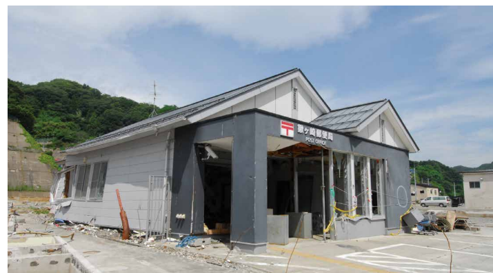
Kuwagasaki Post Office in Miyako City, Iwate Prefecture The tsunami collided directly with the front of the post office. The slant of the walls shows how the water escaped from the building.
